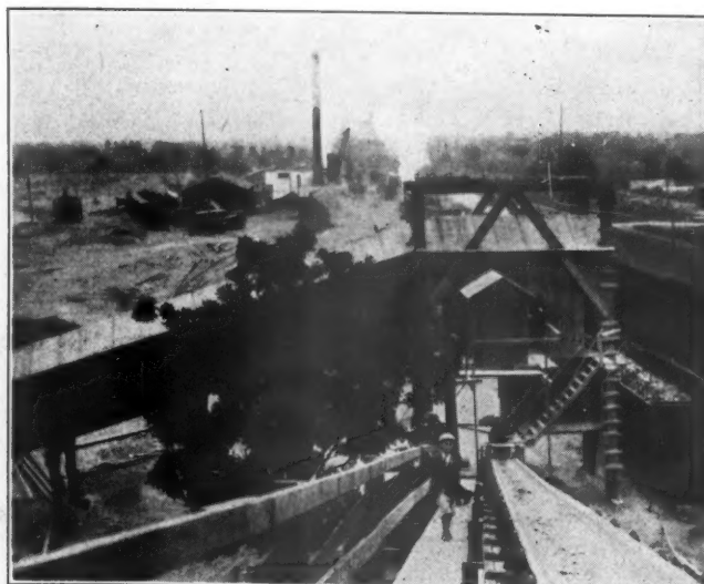
One of the Main Belt Conveyor Units
